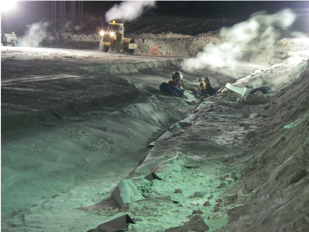
Photo 9: Workers cleaning the frozen core and the GCL liner near Sta. 1+40. Photo looking north from Sta. 1+00.
