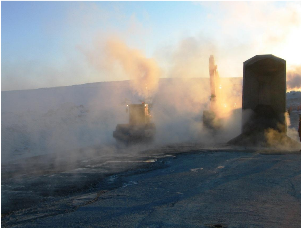
Photo 10: Today's frozen core placement. A sheen was consistently present on the surface. Steam caused poor visibility from the excavator cab.
