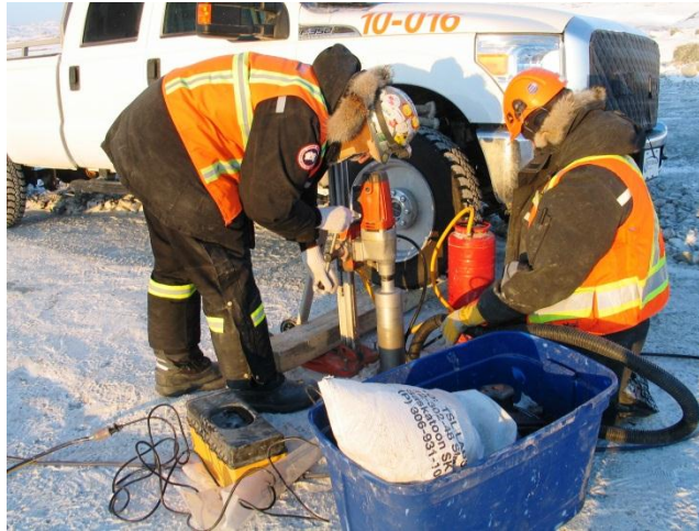
Photos 6: SRK and EBA drilling cores at the dam.
